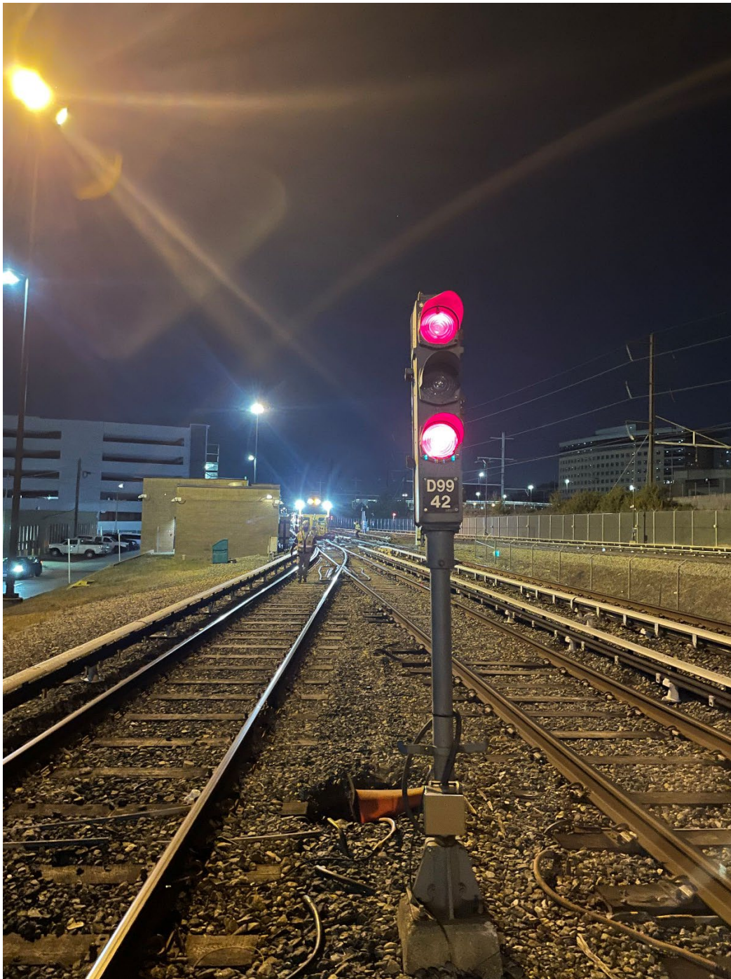
Image 5 – D99-42 Signal displaying a red aspect in the New Carrollton Yard.
