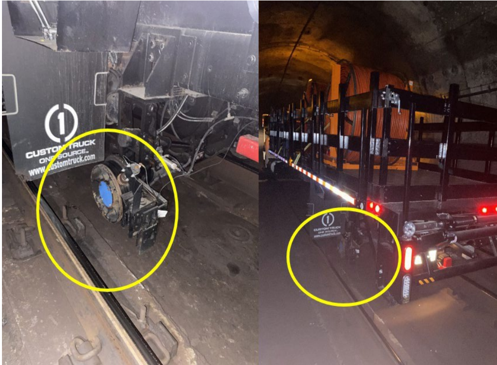
Images 5 and 6 - Depicts the derailed left rear wheel of Hi- Rail Vehicle 9042. (Rear view)
