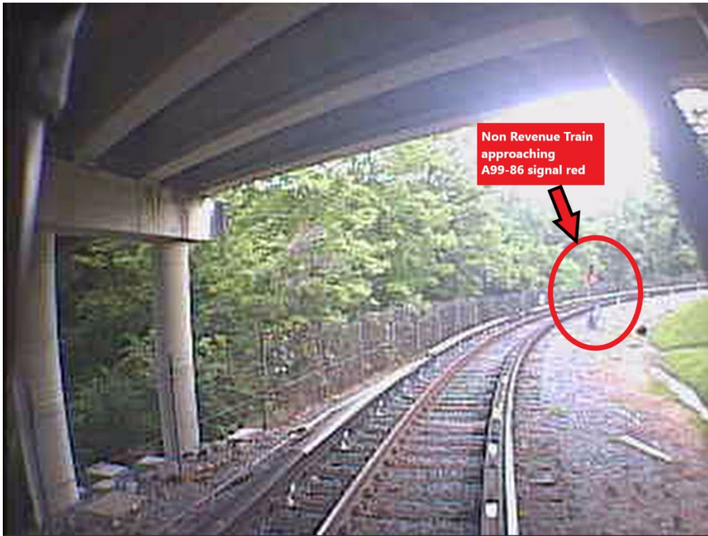
Figure 8 - Railcar 7158 front-facing camera of approach to A99-86 Signal
