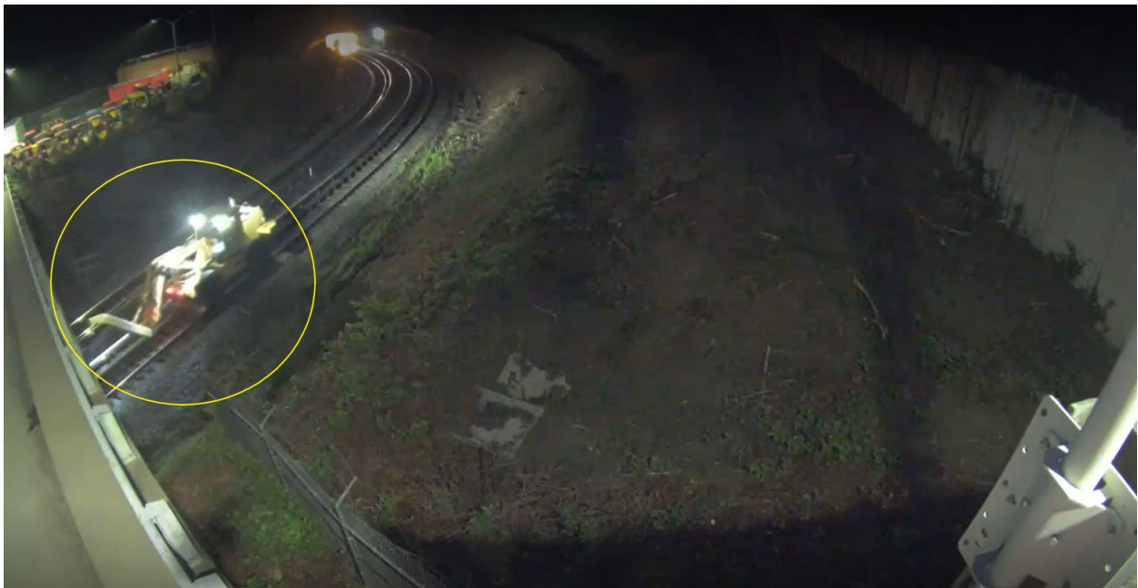
Figure 5 –The WMATA re-railing equipment arrived on the scene at 05:10 hours on YL 1.
