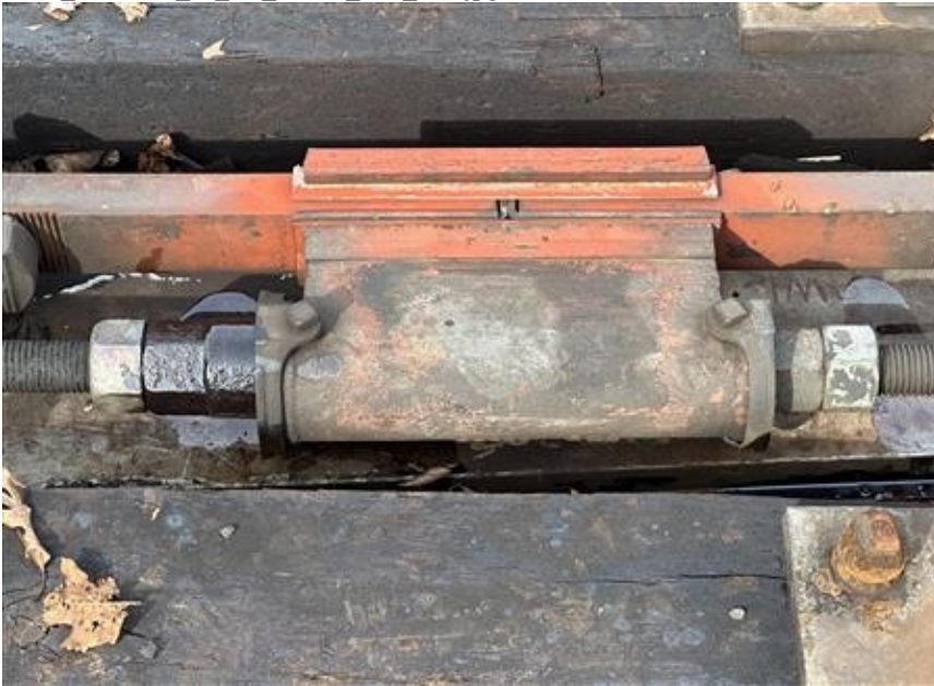
Good insulation on OP Basket Rod B98.jpg
