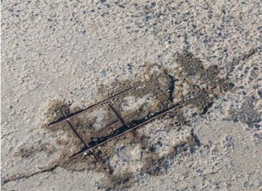
Deteriorating_surface_A99_Shady_Grove_Rail_Yard_061424_lp_3_rp_.jpg
