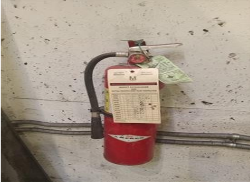
Fire Extinguisher Out of Compliance A99 Shady Grove Rail Yard S and I Shop 061424 lp 1 rp .jpeg
