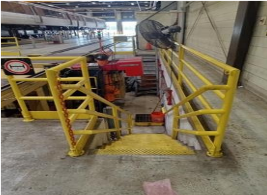
Open_access_hazard_to_wheel_lathe_area_A99_Shady_Grove_Rail_Yard_061424__lp_1_rp_.jpg
