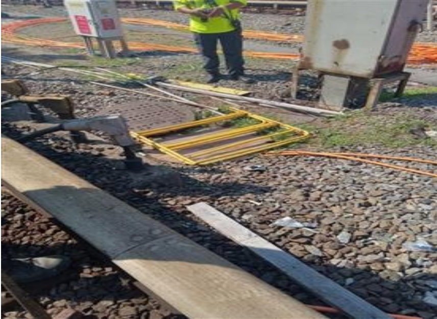
IT barriers on track 2 missing with two out of four red e mn flares not functioning __lp_ACS_rp__061824.jpg
