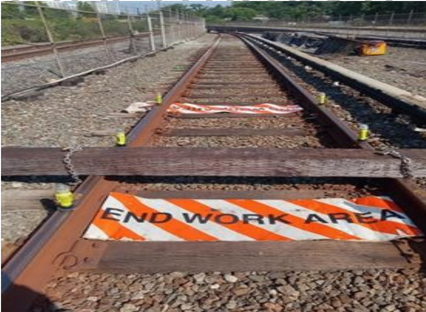
IT barriers on track 2 missing with two out of four red e mn flares not functioning __lp_ACS_rp__061824.jpg
