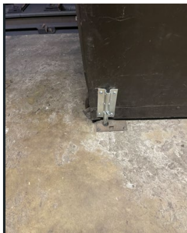
U St AC Room 106 – Door Repaired (picture provided by Metrorail)
