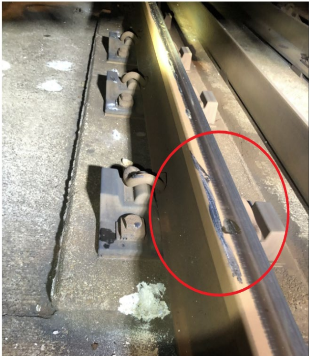
Image 4: Shows the Point of Derailment.
