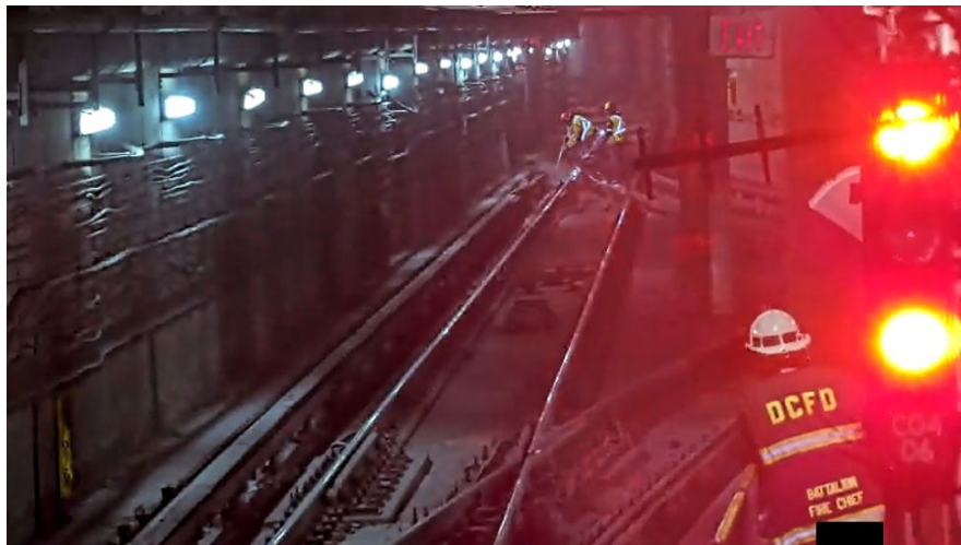
Figure 6 - depicts ERT clearing the debris from the roadway as DCFEMS remains within the confines of the continuous handrail.
