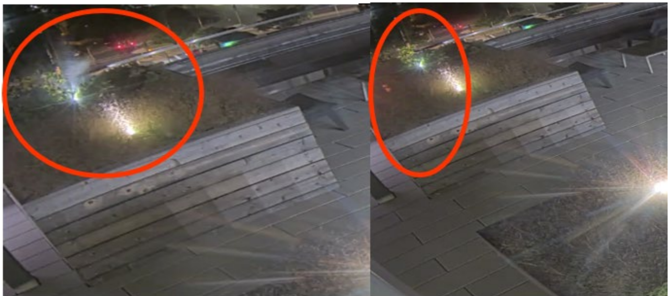
Image 5 – Images of smoke and then fire beginning to burn within the wooden flower planter.
