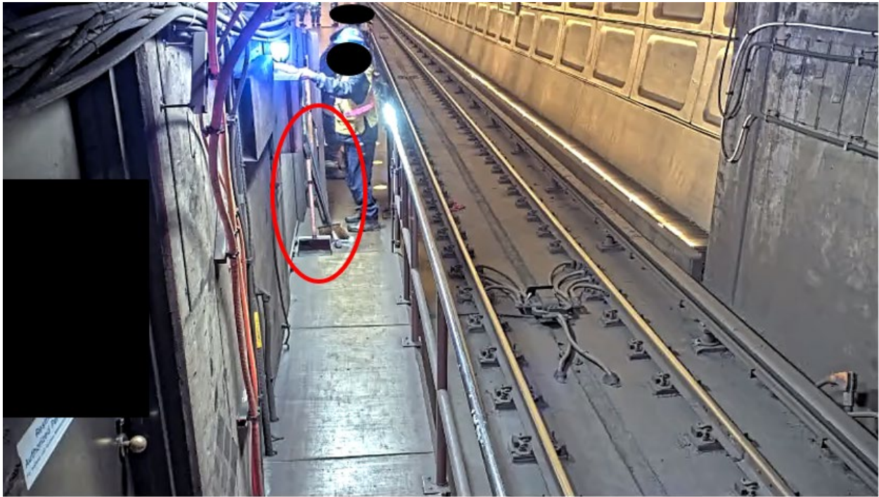
Figure 17 - ERT personnel obtaining equipment to clear debris in the roadway.
