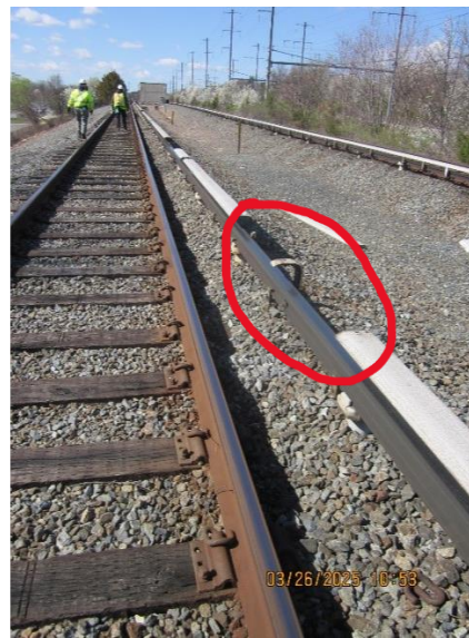
Fig 13 and 14 - more damaged or removed third rail coverboards.
