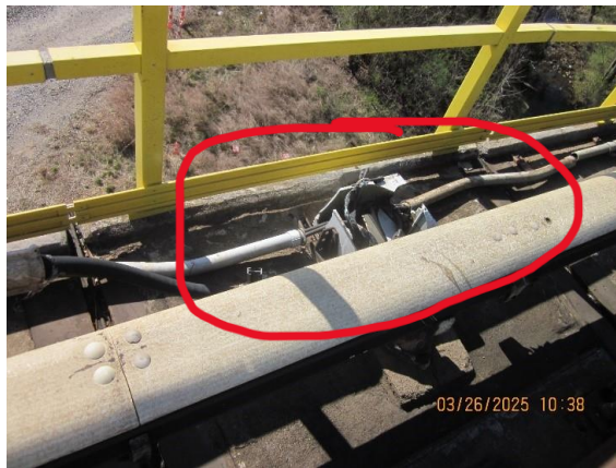
Fig 3 and 4 – damaged junction box and chain marker
