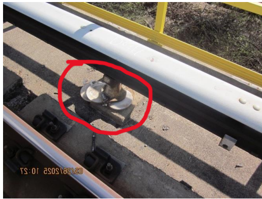
Fig 7 and 8 – detached shims
