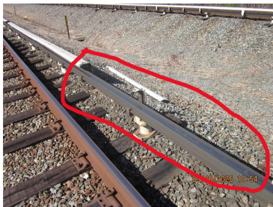
Fig 13 and 14 - more damaged or removed third rail coverboards.
