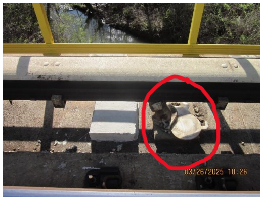
Fig 5 and 6 – shims detached from under the insulators
