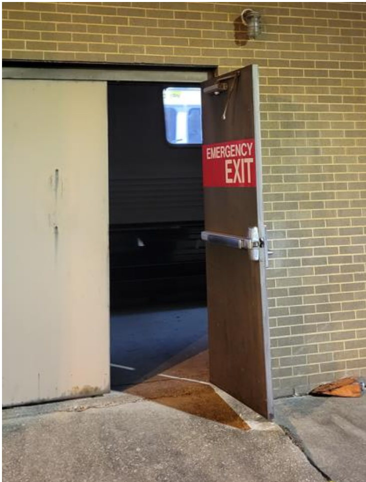
Fig 3 – open and broken emergency door – wide angle
