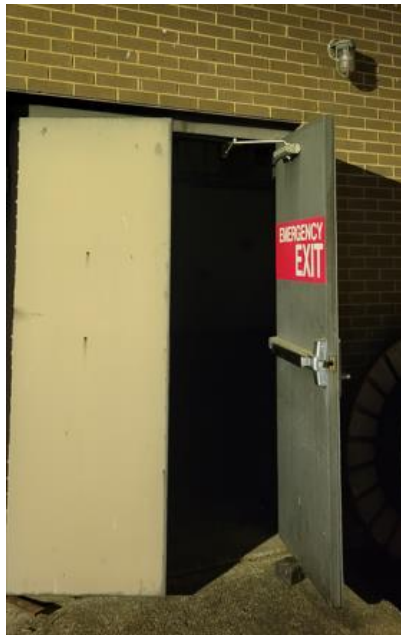
Fig 1 – open wedged emergency door
