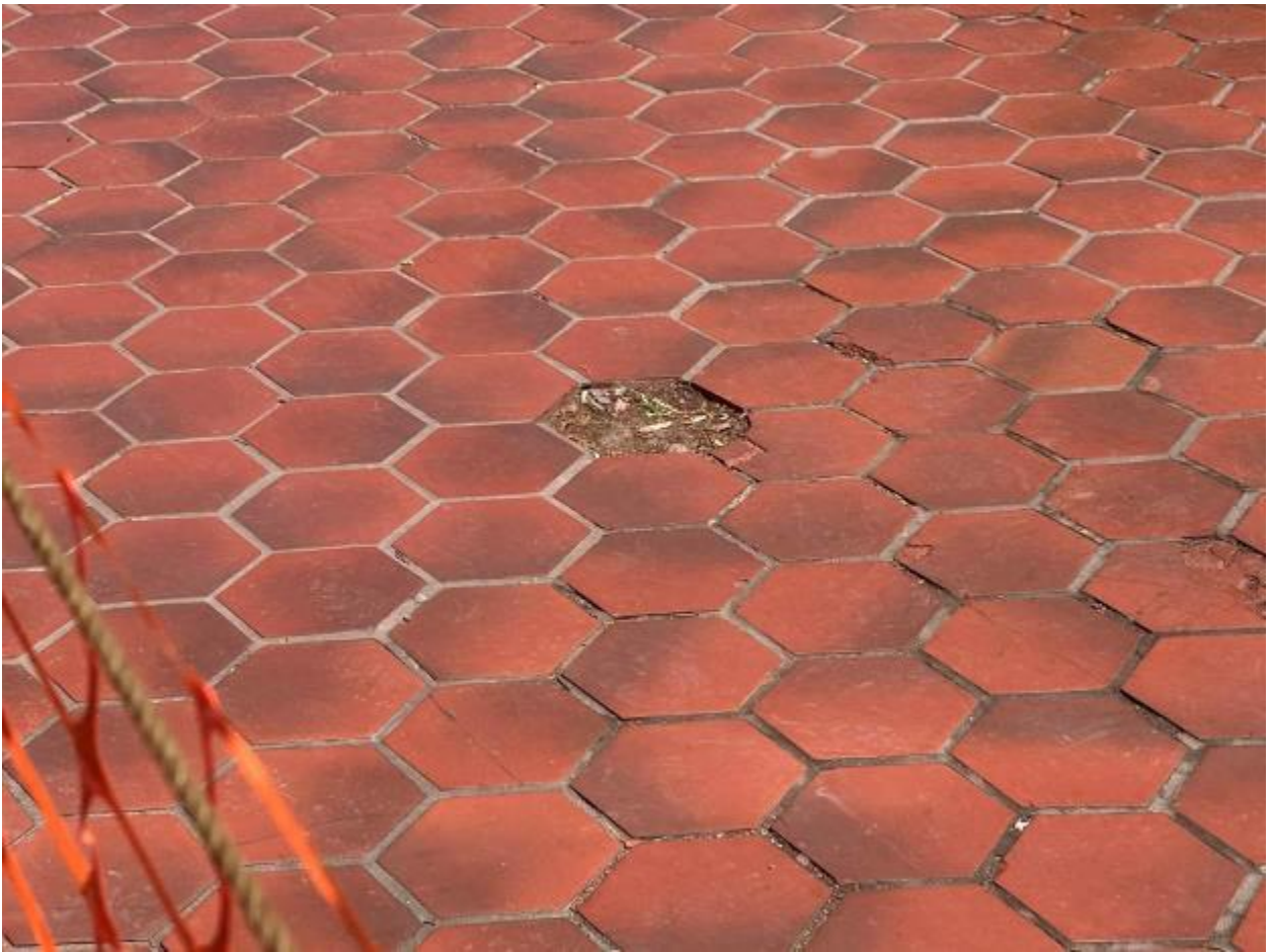
Fig 4 - missing tile
