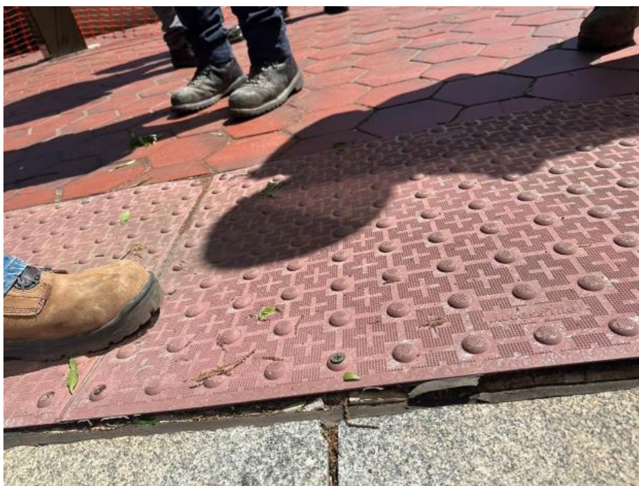
Fig 1 Tilt of granite edge, gap between granite and ADA warning tiles
