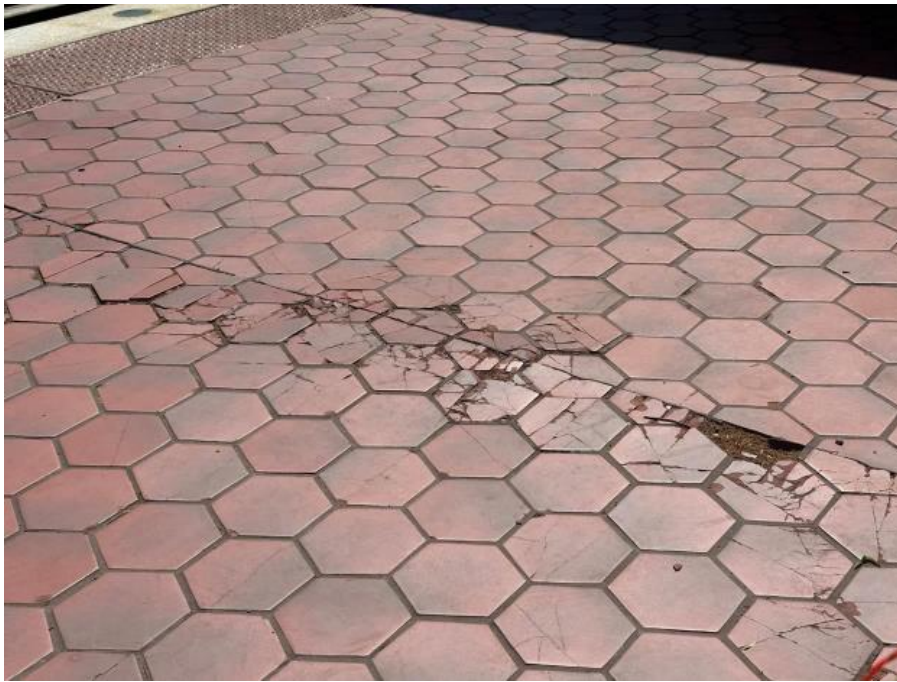
Fig 2 Loose and broken tiles
