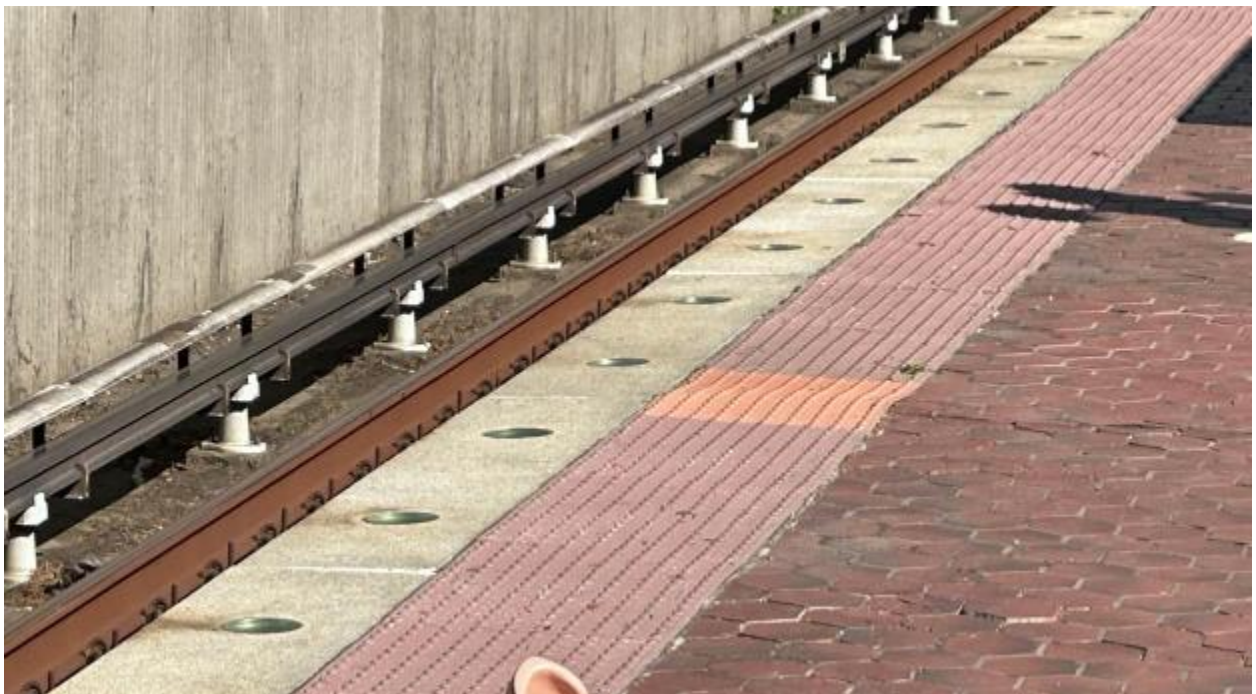
Fig 3 Buckled ADA warning tile
