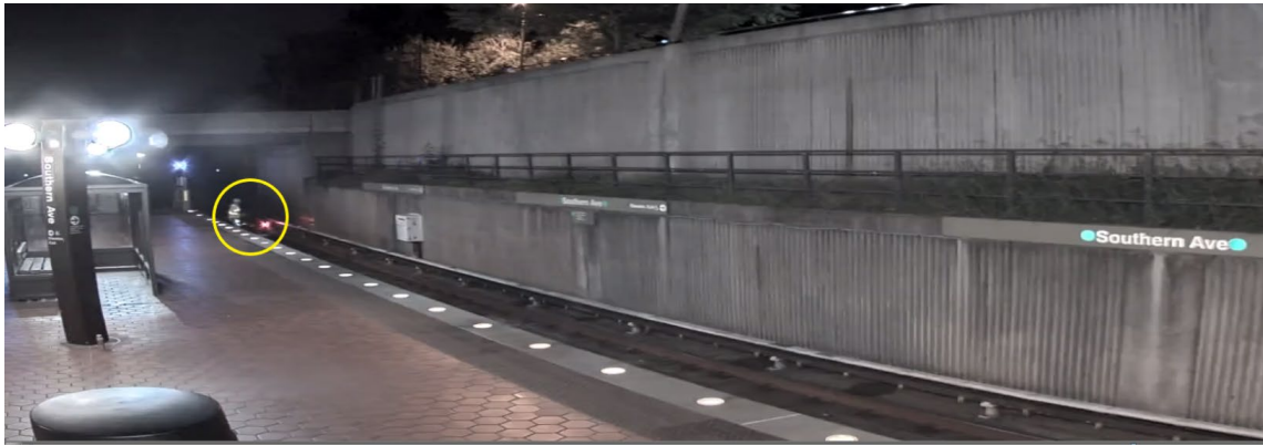
Figure 6 - depicts the RWIC placing a shunt on Track 2 at Southern Avenue Station at 02:13 hours.
