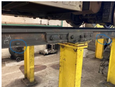
Photo 1: Showing the missing bonding return cable and the installed bonding cable on track 2N
