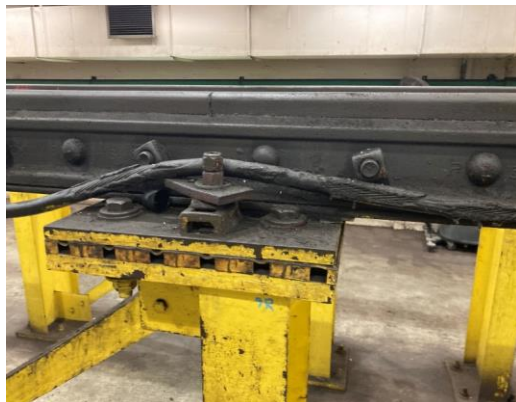
Photo 2: Bonding cable with insulated cover showing deterioration and replacement bonding cable on track 3N.
