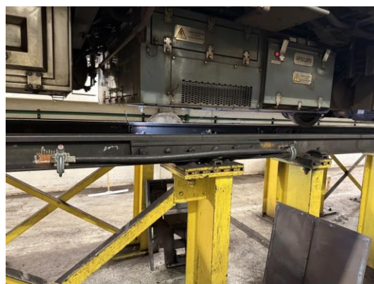
Photo 2: Bonding cable with insulated cover showing deterioration and replacement bonding cable on track 3N.
