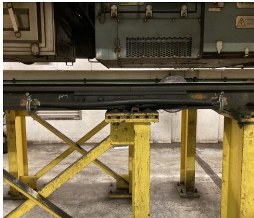
Photo 5: Replacement of third missing cable on track 3N
