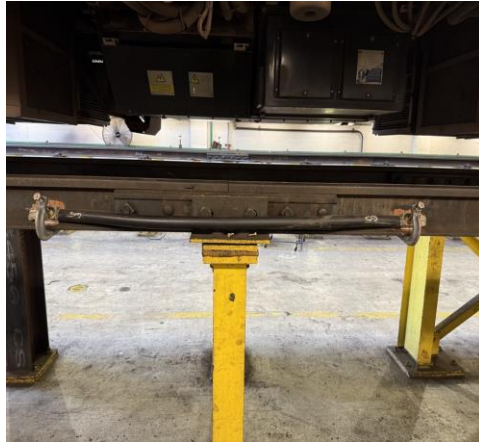
Photo 4: Replacement of second missing cable on track 3N
