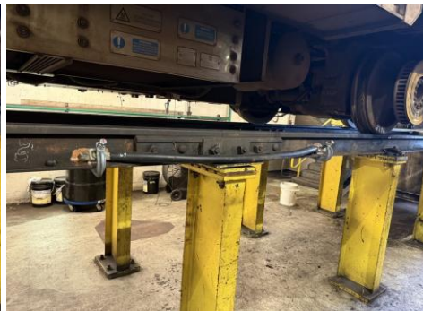
Photo 1: Showing the missing bonding return cable and the installed bonding cable on track 2N
