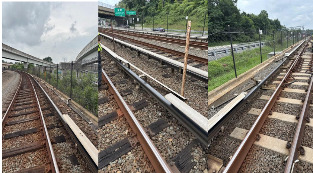
Photo 6 (left). Missing cover boards.
