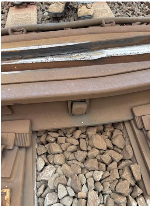
Photo 5. The loose middle frog bolt contributes to wear on the frog and causes banging. Because the frog is at the convergence of two lines, replacement and tamping are recommended due to the wear stated in the TRST-1000 section 108.6 (F).
