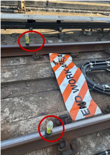
Photo 6. Red lanterns were not illuminated. Issue was mitigated onsite.
