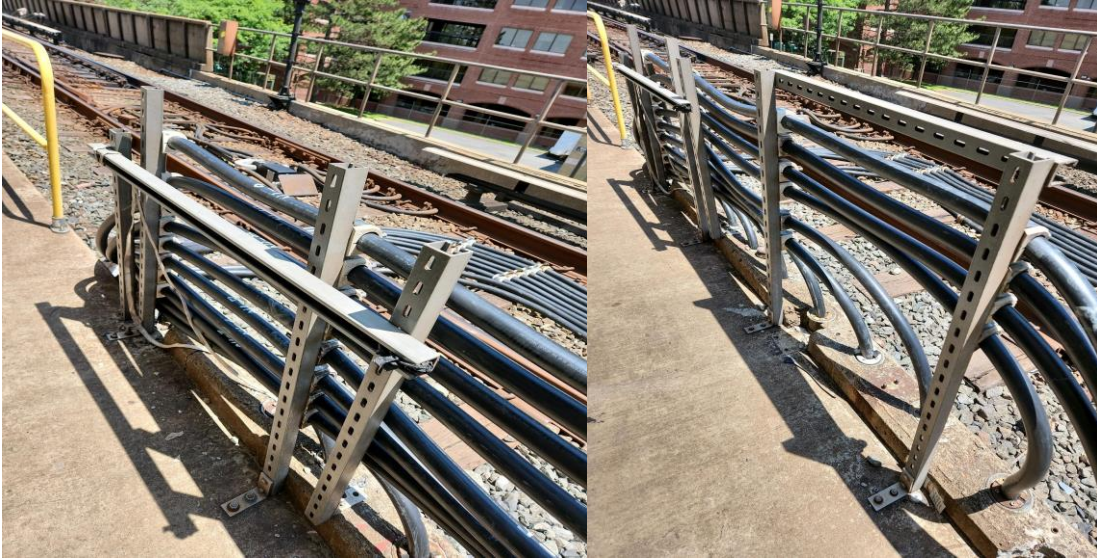
Photo 2 (Left). Structure being held together with discarded polyester webbed pull tape.
