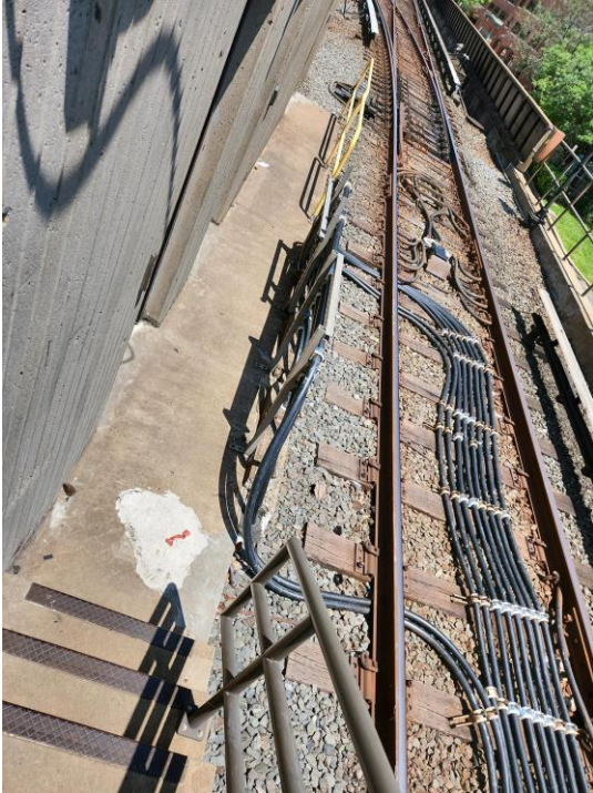
Photo 1. The gap between the handrails exceeds six feet.
