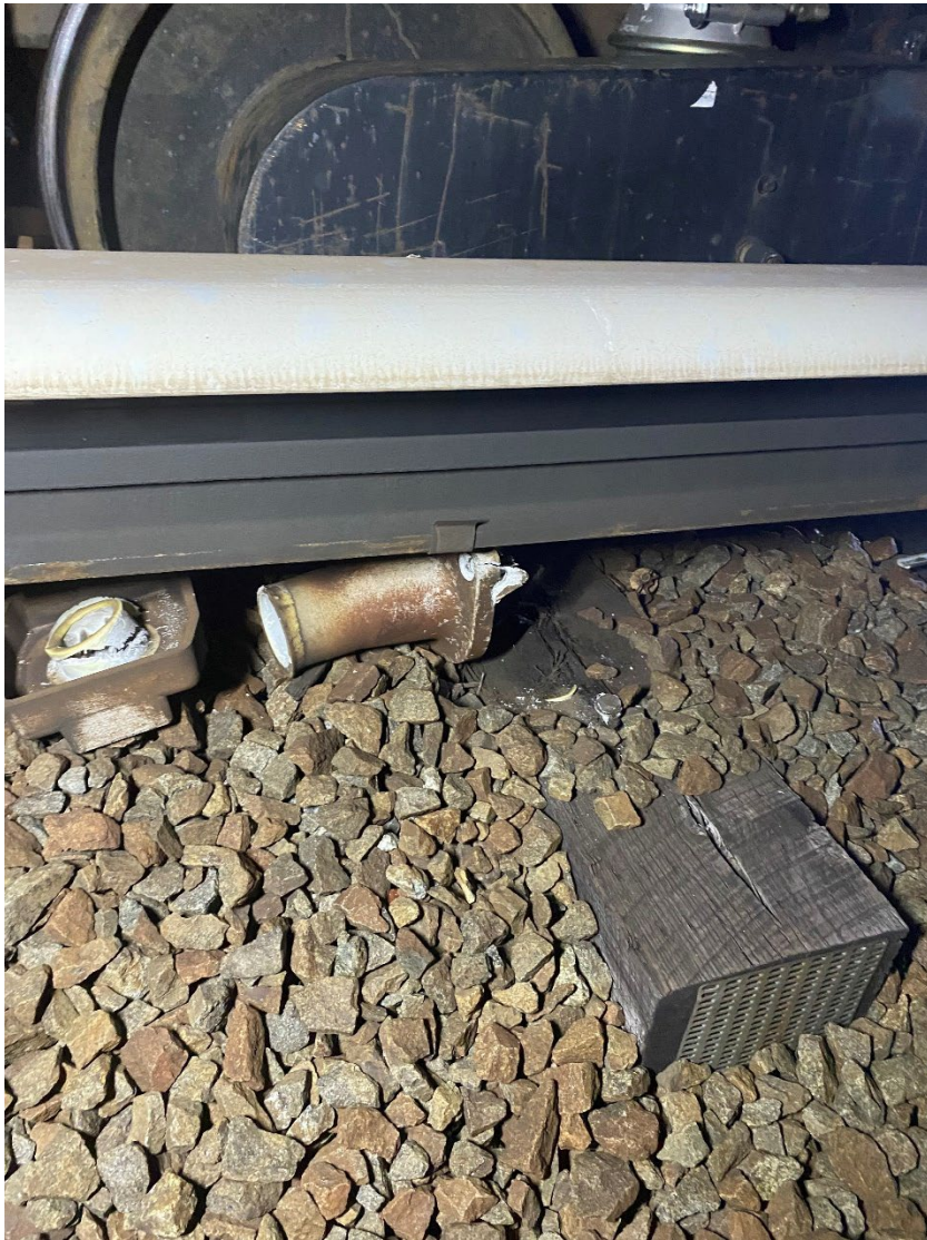
Figure 21 - Depicts damages to the Third Rail insulator.
