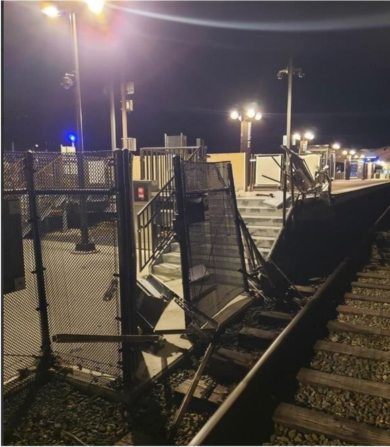
Image 6: Shows damage to the ETS Box and handrail.
