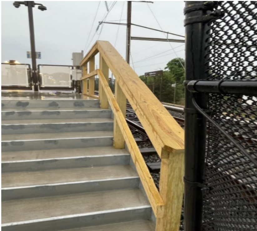
Image 4 - Image 2 of the new ETS Box and temporary wooden railing.
