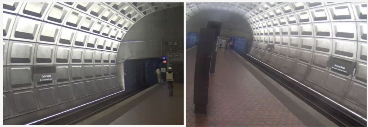
Image 1 - The left image shows the RWIC entering the roadway at Capitol Heights Station, and the right image shows the AMF in place at Benning Road Station 8-car marker.
