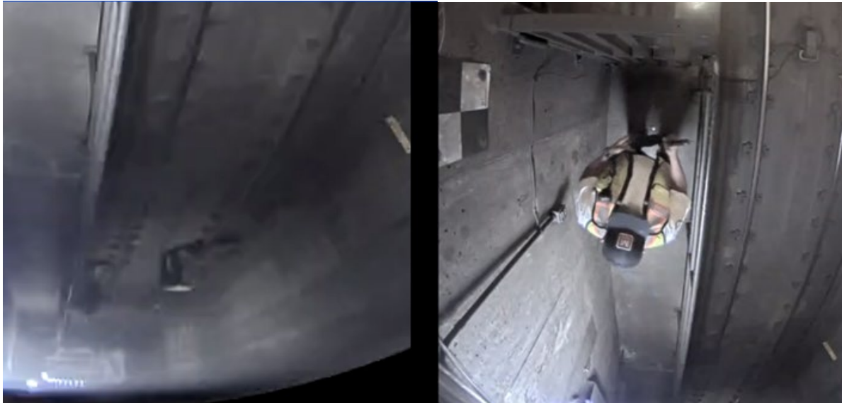
Figure 4 The images above show the RTRA Supervisor hot-sticking and returning to the platform without visible high-voltage gloves.
