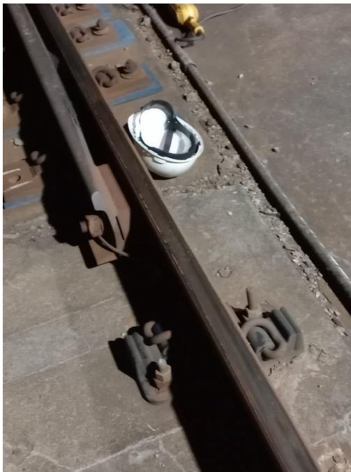
Photo 3: Hard hat not being worn as work was underway.
