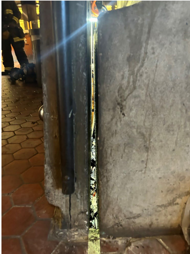
Image 1 – Image of a gap in the parapet wall where debris accumulated.
