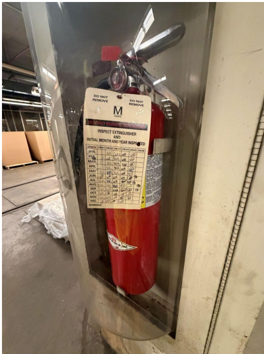
Photo 2: Example of one WFC shop fire extinguisher inspected which was properly maintained and unexpired. All fire extinguishers inspected were found to be in this condition.
