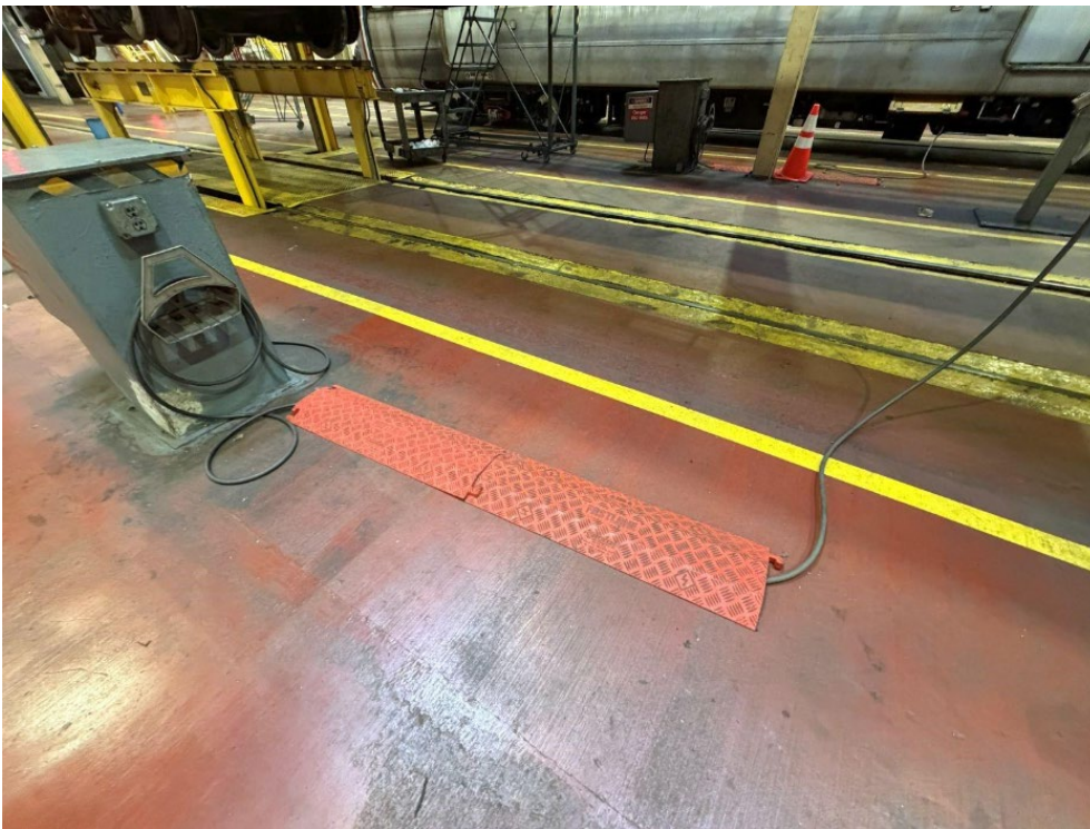
Photo 8: Properly covered high voltage cables.
