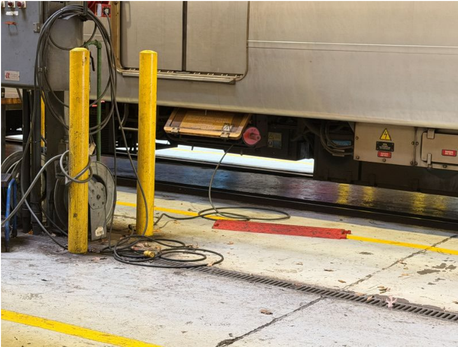
Photo 6: Uncovered power cables at Greenbelt (E99).
