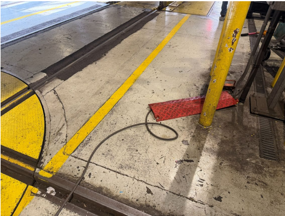
Photo 7: Uncovered power cables at Greenbelt (E99).
