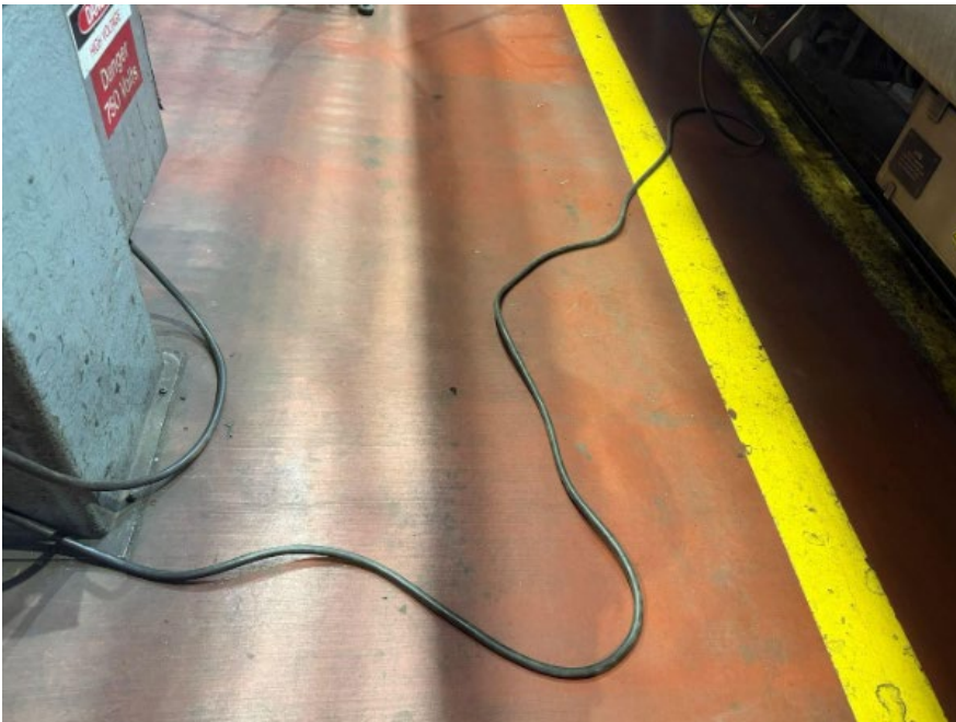
Photo 10: The one area of exposed high voltage cable wires that were not covered but was mitigated onsite.
