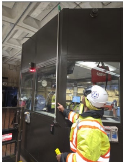
Photo 4: Unsecured metal pole used to retrieve fallen items at Dupont Circle (A03).
