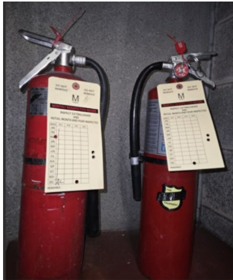
Photo 8: Fire extinguisher (right) missing inspection signatures in fire equipment cabinet 101 in room RMC-200 at Woody Park (A04).
