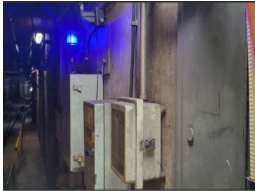
Photo 3: An example of a mitigated legacy non-operational ETS box that was sealed shut at Judiciary Square (B02).
