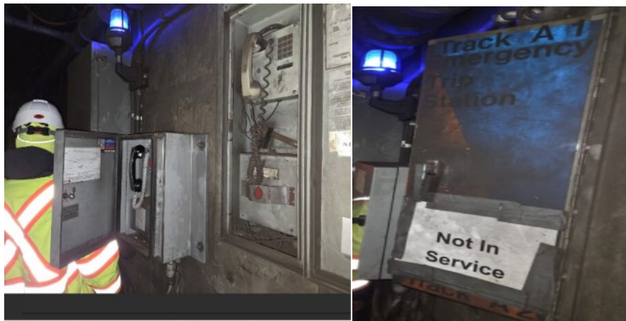
Photo 1 (left): An open non-operational ETS box at Farragut North (A2).
