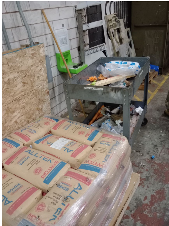
Photo 6: Blocked Eye Wash Station.
