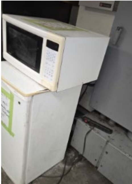
Photo 31: Appliances not directly plugged into the wall outlet.
