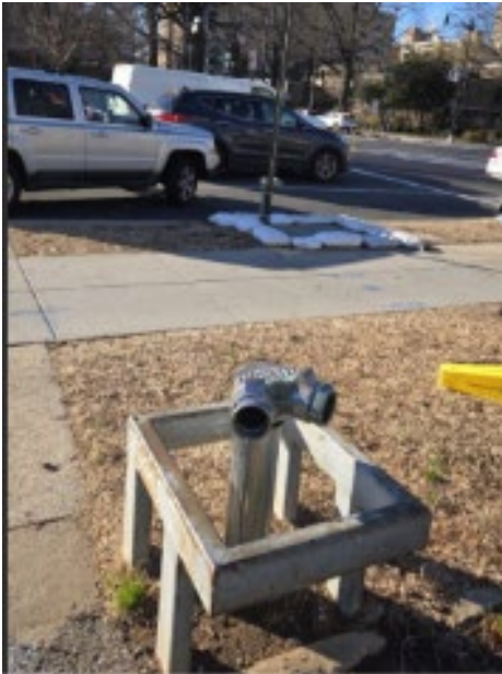
Photo 32: Standpipe missing protective covers.
