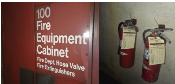
Photos 19 (left) and 20 (right): The cabinet with the expired fire extinguishers. The past due extinguishers themselves.
