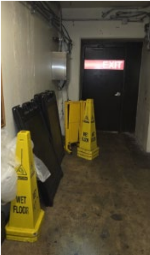
Photo 3: Partially blocked Exit door.
