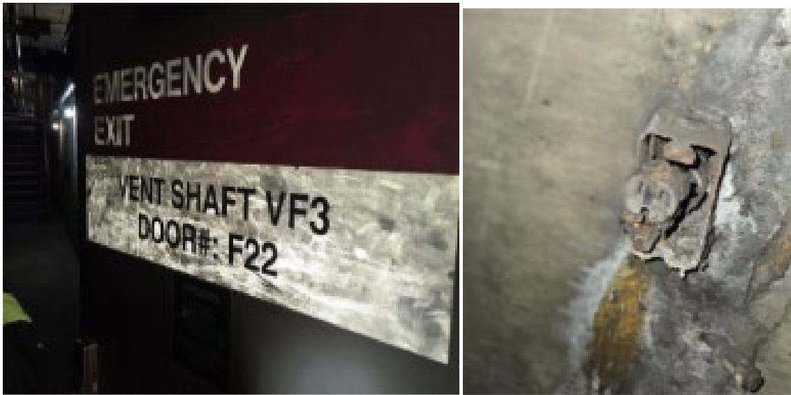
Photos 12 (left) and 13 (right): Electrical outlet. Plus IFC 604.6 – Unapproved conditions.
