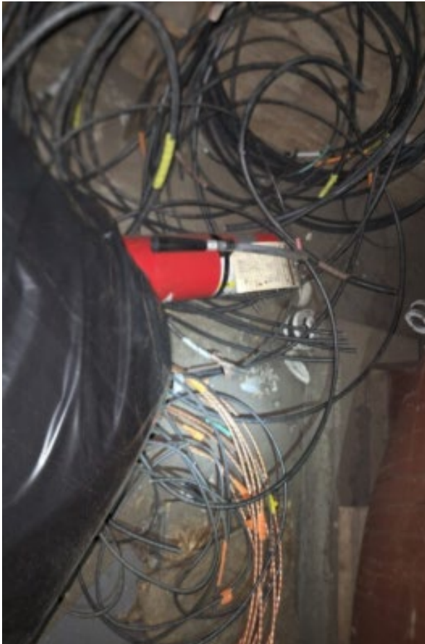
Photo 11: Debris in room and fire extinguishers not mounted.
