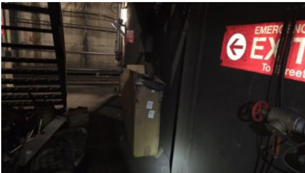
Photo 15: Combustible storage is not permitted in exits, stairways, or ramps.
