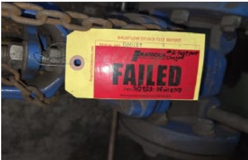
Photo 4: Failed Backflow Protection Valve.
