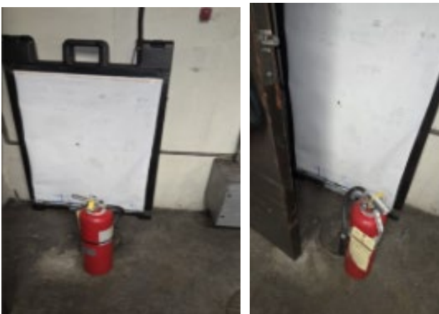
Photos 29 (left) and 30 (right): Portable fire extinguisher on floor.
