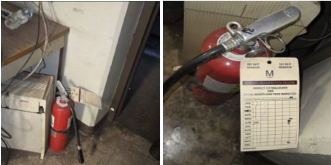
Photo 8 (left) and photo 9 (right): Fire extinguisher not mounted and past its monthly inspection.
