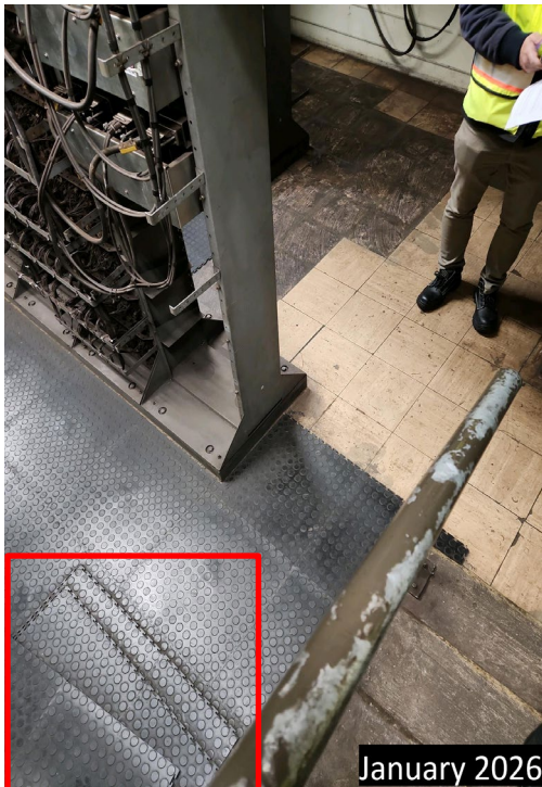
Photo 4: 2025 Metro Center Station (A01) Missing TCR flooring in January 2026.
