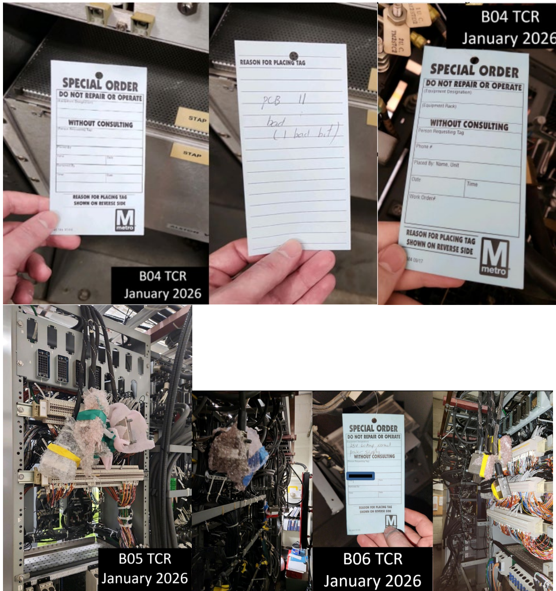
Photos 5 to 9: Improper blue tagging.
