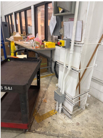
Photo 11: A movable cart blocking the emergency button to stop stinger electrification.
