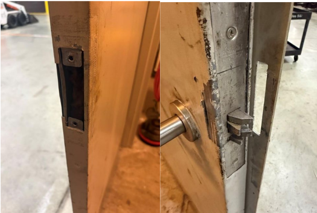
Photos 16 (left) and 17 (right): Unsecured Grease Room double door.
