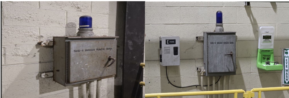
Photos 2 (left) and 3 (right): two of the three ETS boxes without blue lights illuminated.
