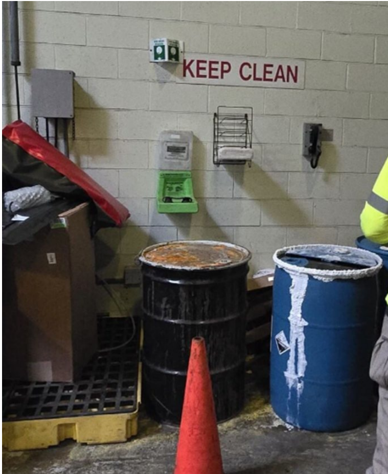
Photo 7: Obstructed access to eye wash station. (See Defect 6 for more information regarding the chemical container hazard.)
