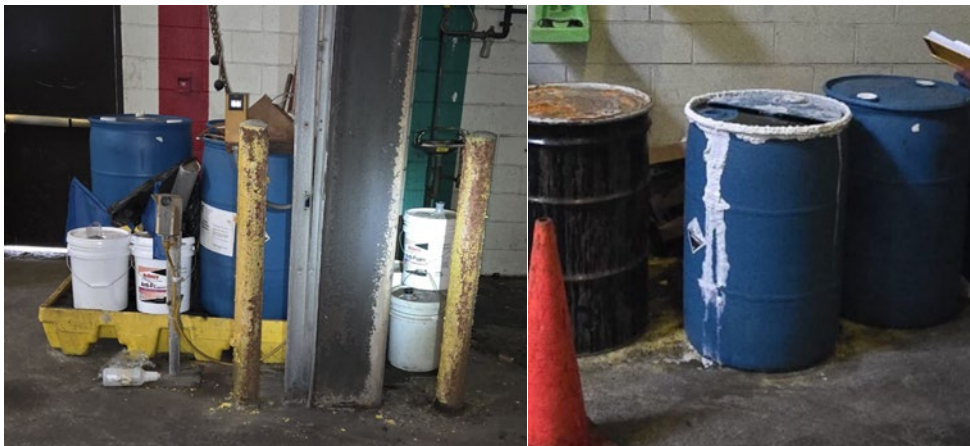
Photos 10 and 11: Improper chemical storage with leaking exposure hazard.
