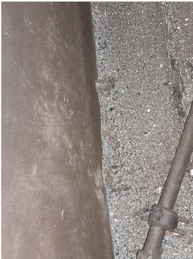
Figure 19 - A pipe on the ground.
