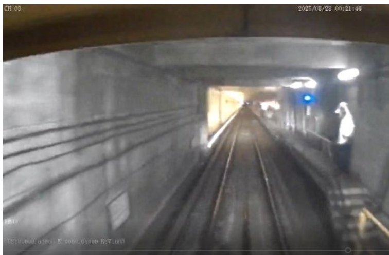
Figure 18 Screenshot from PM46's front camera of PM46 passing the second roadway worker in a place of safety.
