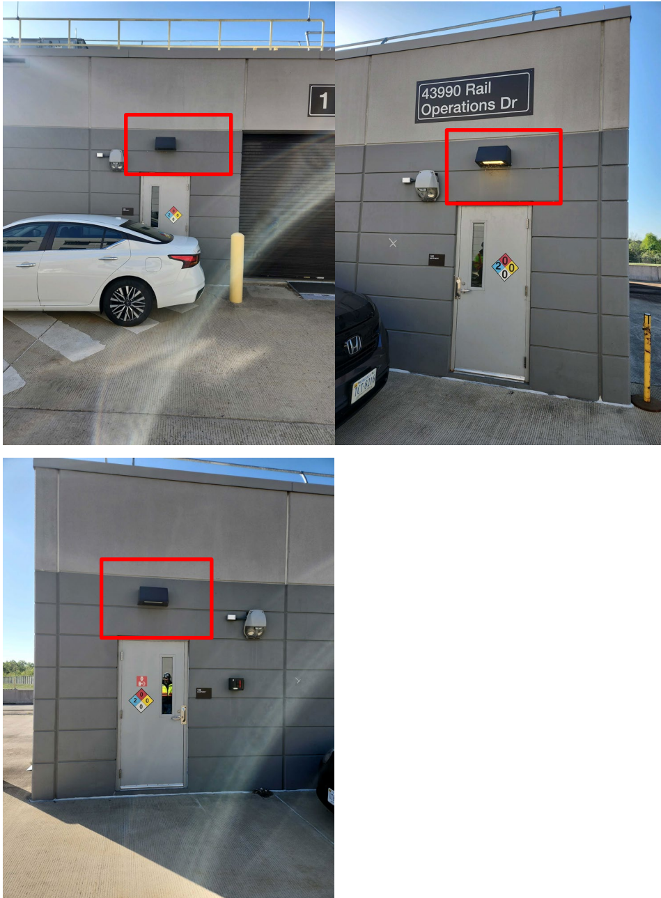
Photos 1-3: Direct access to the Dulles Yard (N99) car wash with no warning system that a train may be transiting through the wash when entering the facility via these doorways.
