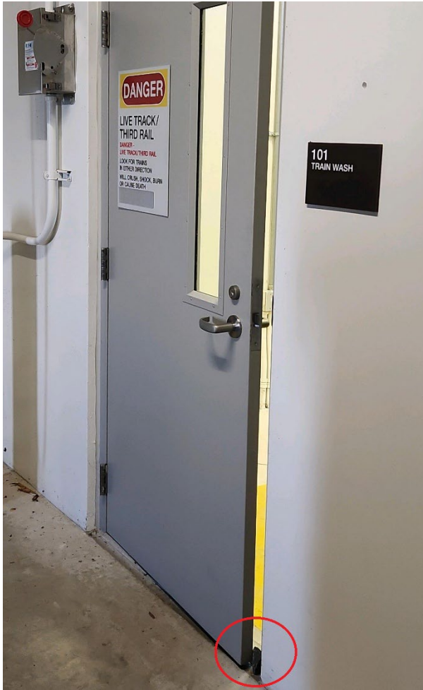
Photo 6: Door propped open that should remain secured and closed because of hazards on other side.
