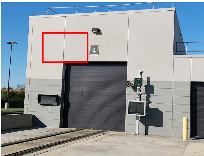
Photo 8: Entrance (facing east).
