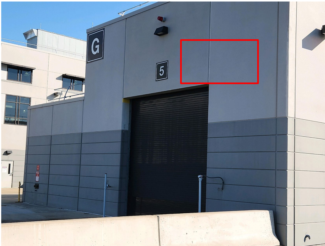
Photo 10: Exit (facing west).
