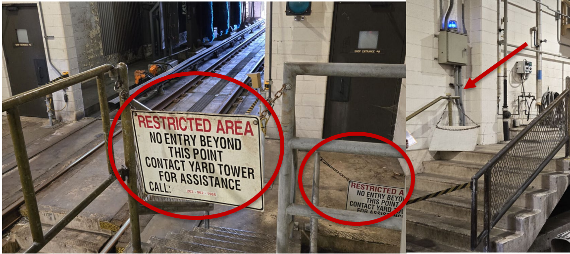
Photos 5 (left) and 6 (right): example of two signs that were able to be reattached and the area where the one sign's chain is not long enough for a reattachment of the warning sign.
