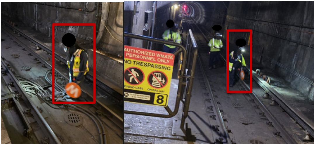
Photos 4 (right) and 5 (left): Left – At Cleveland Park Station (A05) , the watchperson conducting roadworker duties while functioning as the sole watchperson for the work crew. Right – the work crew walking track and fouling the roadway.
