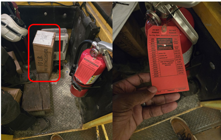
Photos 2 (left) and 3 (right): The new unboxed fire extinguisher and the missing expiration date on the prime fire extinguisher inspection tag.
