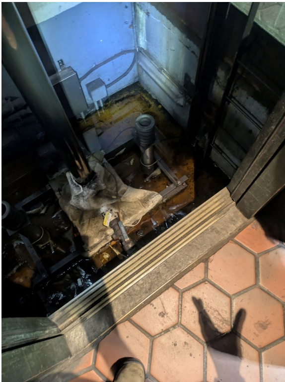
Photo 2: Overall view of the pit of elevator #1.
