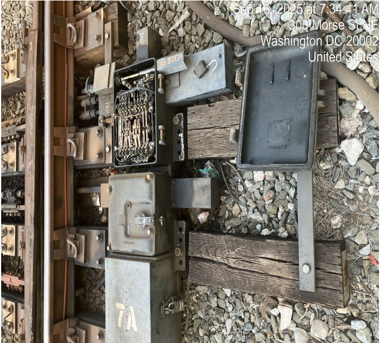
Image 3: Depicts Signals Maintenance inspections of the switch machine 7A.
