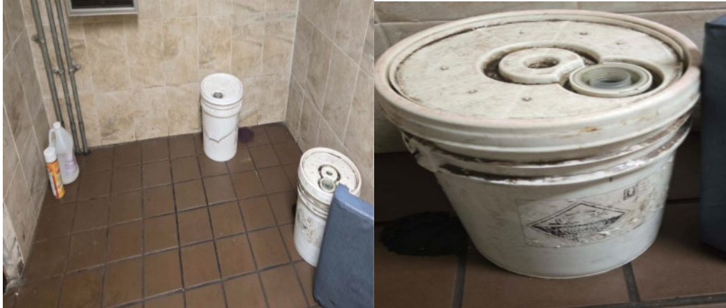
Photos 18 and 19. Chemicals stored in the employee bathroom.
