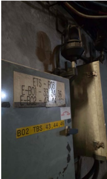
Photo 8. ETS blue light B-03 is not illuminated.
