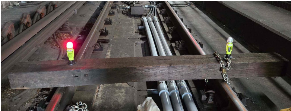
Photo 5: Wood tie only secured with one lock.
