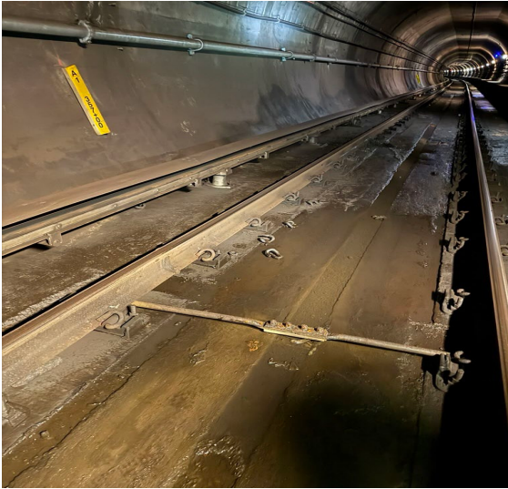
Photo 1: Existing gauge rod at A1 357+00.
