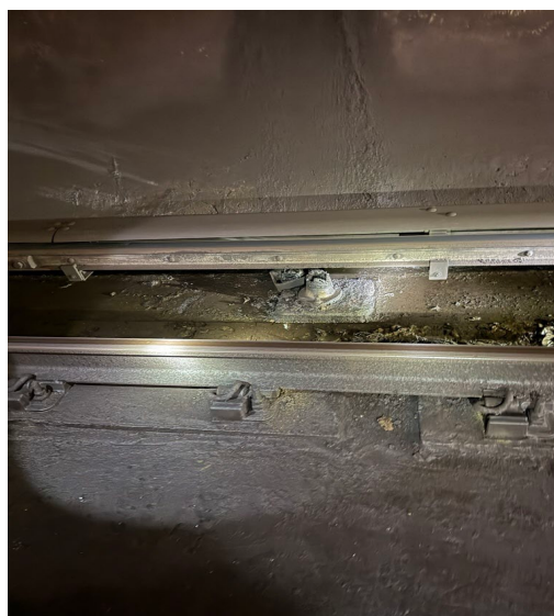
Photos 2 (left) and 3 (right): Show broken third rail insulators.
