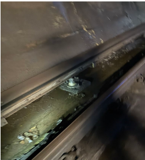
Photos 2 (left) and 3 (right): Show broken third rail insulators.
