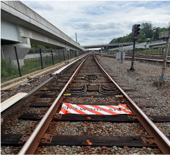
Photo 6: Shows the setup for exclusive track occupancy setup with work mat, e-flares (flashing as required), and shunts in proper position.
