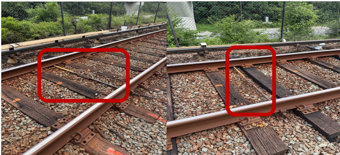
Photo 1 (left) and Photo 2 (right): Photo 1 shows the installed gauge rod at K2 512+90. Photo 2 shows the installed gauge rod at K2 513+90.
