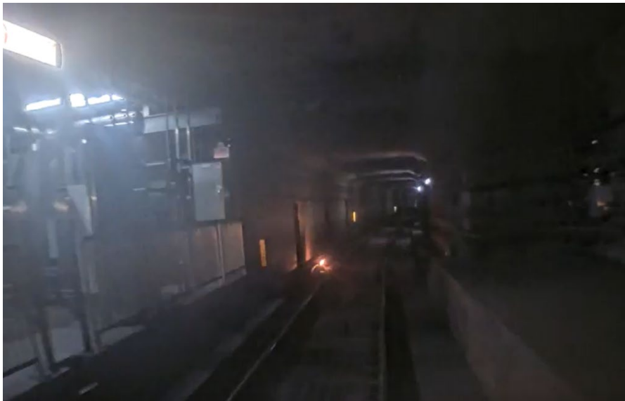
Picture 4 – Depicts the forward-facing camera and RVO'S Point-Of-View on approach to the reported fire, part 2.
