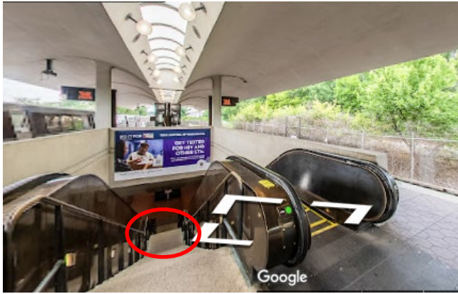
Figure 1: Shows the staircase landing at Shady Grove Station where the customer was found after falling down the stairs.
