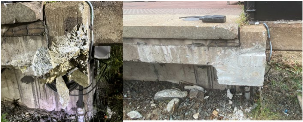
Image 3 – Before and after repairs photos of the concrete area beneath the platform.
