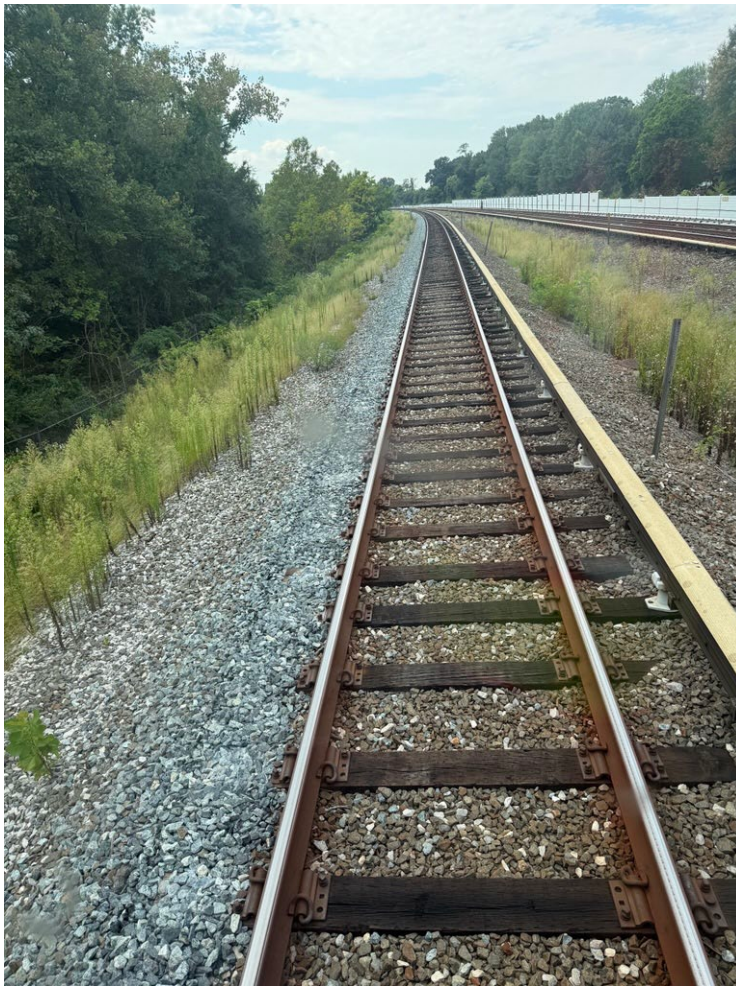
Photo 3: Shows new ballast mitigation on the shoulders of the ties between College Park (E09) and Greenbelt (E10).
