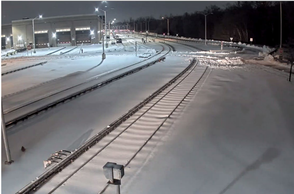
Image 1: Depicts yard lead track conditions before the derailment.
