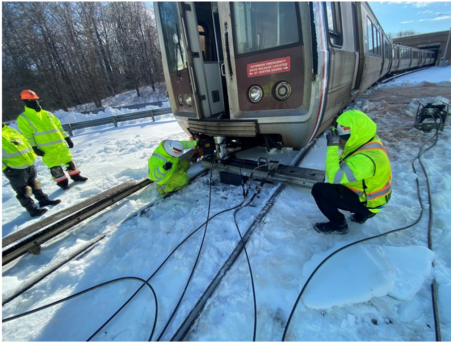
Image 5: Shows CMNT re-railing Train ID 805.
