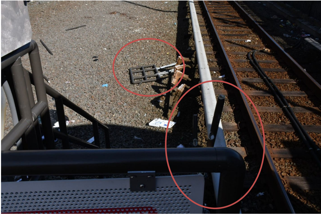
Image 5 - Closer view of damaged end gate and railing
