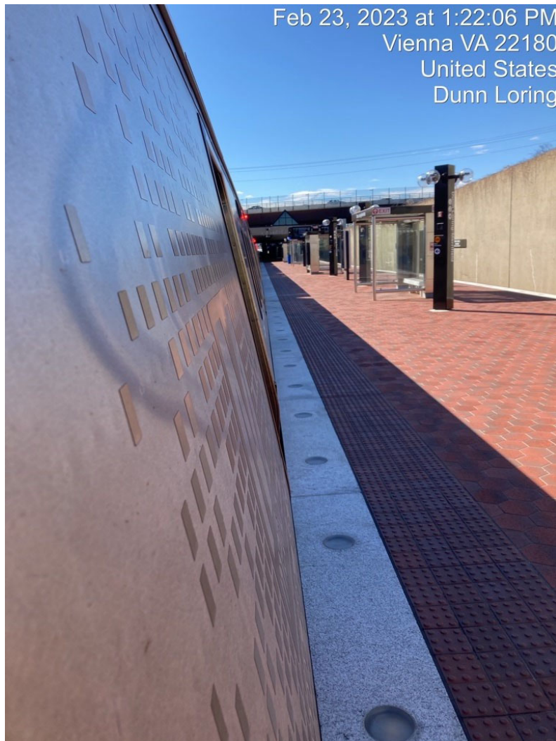
Image 2 - View from the area of the Operator's cab window looking towards the rear of the train. The seventh car is under the station canopy in the shadowed area.
