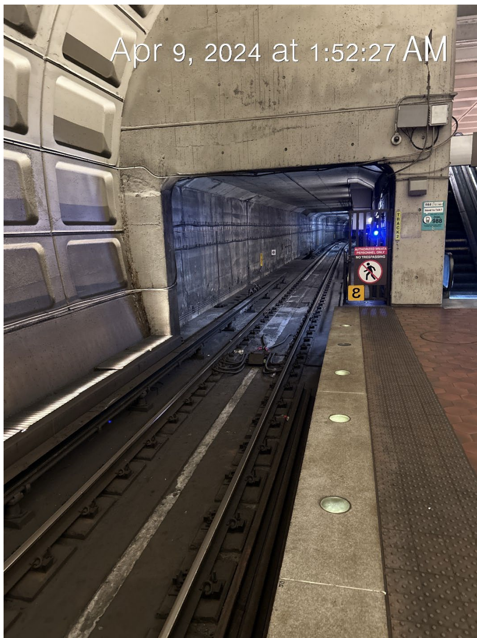
Figure 18 - track 2, Stadium-Armory Station, tunnel view in the direction of the D&G Junction
